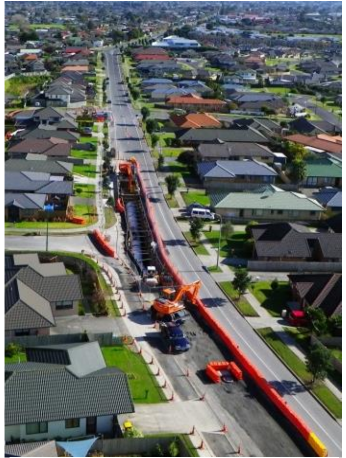
Figure 24: Example construction area with traffic management
