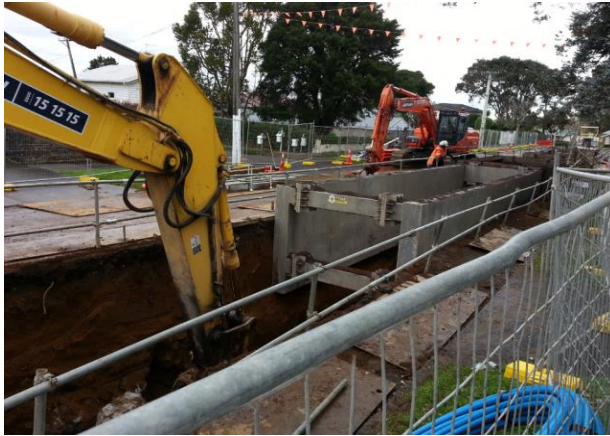
Figure 23: Trench being dug in road reserve
