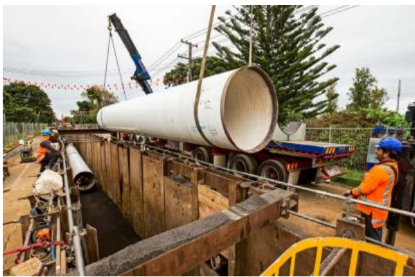
Figure 22: Pipe section being lowered into trench
